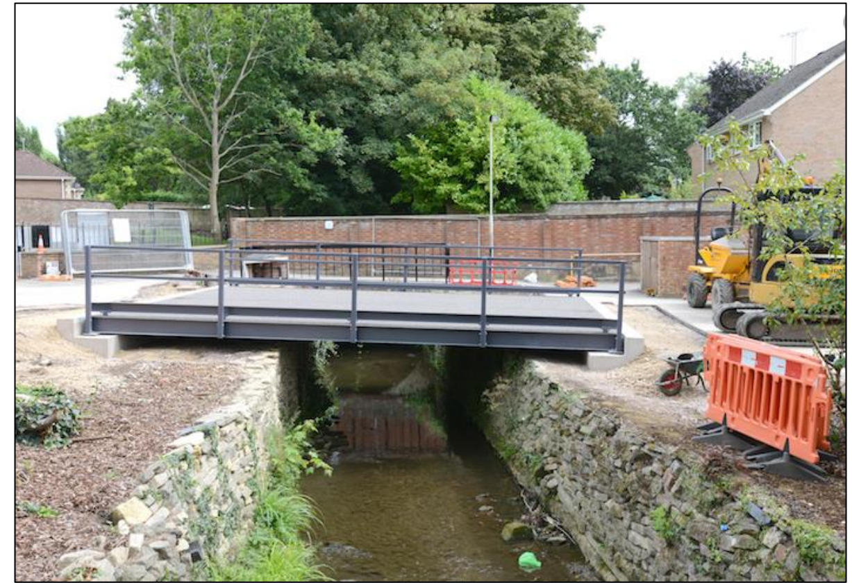
Figure 3.1: Example of temporary span bridge
